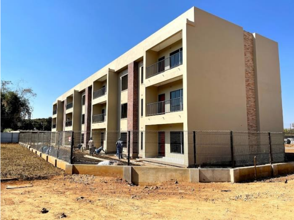
Clear vu fencing in front of the building
