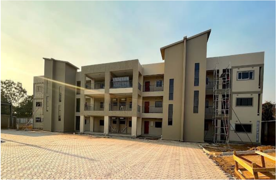
Car park paving
